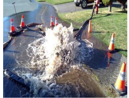
Typical set-up for water hydrant flushing
