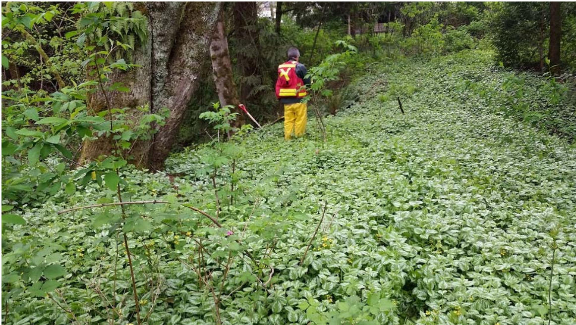
Photo 13. (WP18-FILL/SUMP). Lyncean Creek West (East Tributary). Ravine Fill with High/Low Inlet Culverts
