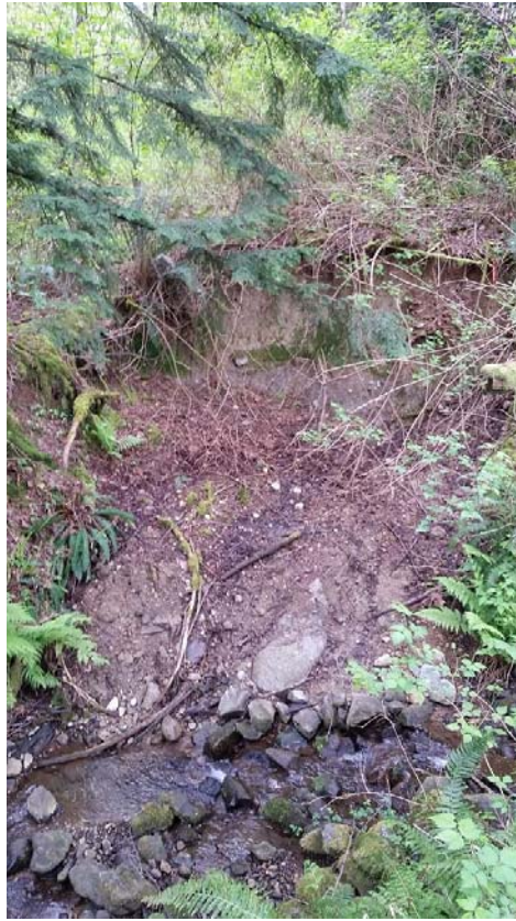
Photo 19. (WP CENTER CREEK). Centre Creek. Right Bank erosion and slide scar (~15m 3 ). Age of event ~5-10 yrs
