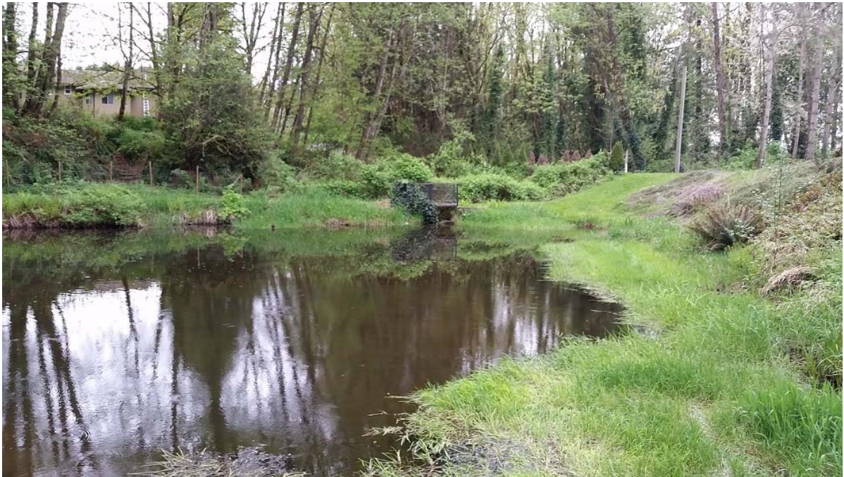
Photo 7. (WP20-POND). Leoran Brook (middle section). View of man-made pond. Outfall wiew with fish ladder structure visible at centre of image.
