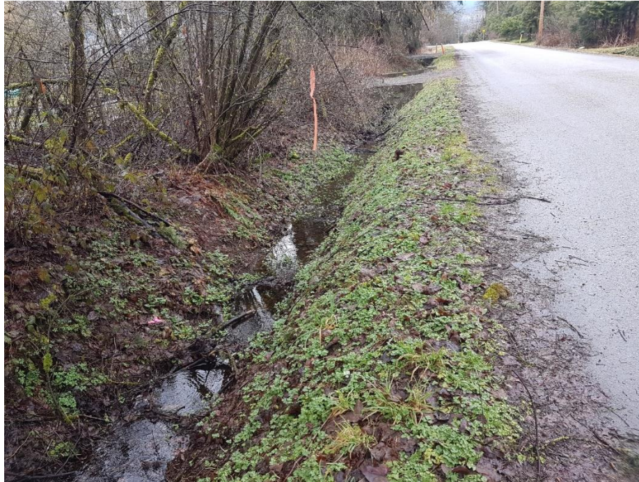
Photo 12: Ditch D3, an example of a typical Class B watercourse with channel definition and riparian vegetation that is likely a source of food and nutrients to downstream fish habitat.
