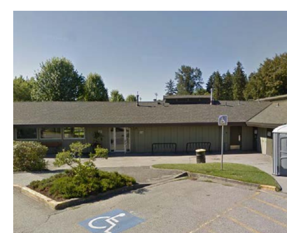
4 North Surrey Minor Football Pavilion
