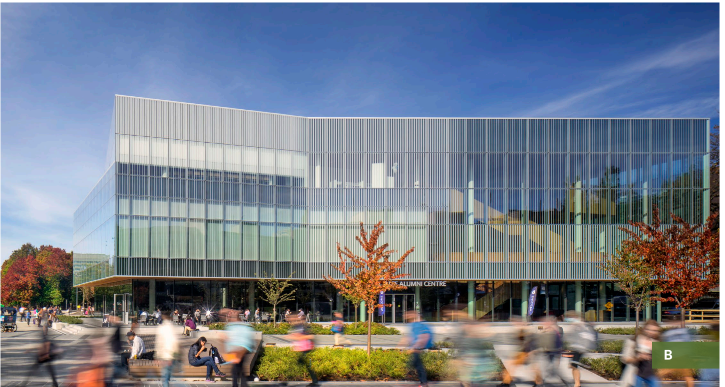
A - Exterior shielded lighting - User controls direction, intensity and duration of lighting - Credit: Selux B - Robert H. Lee Alumni Building - Credit: Nic Lehoux Architects: KPMB Architects in joint venture with HCMA Architecture + Design
