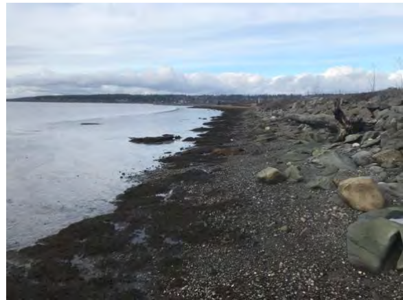
Figure 11 Narrow gravel beach in front of armored dike
