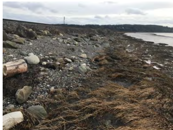
Figure 12 Rock armored with vegetated bench
