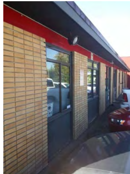
Stacked Bond on Rear Facade
