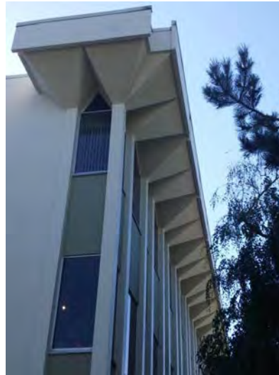
Concrete Cornice: Surrey
