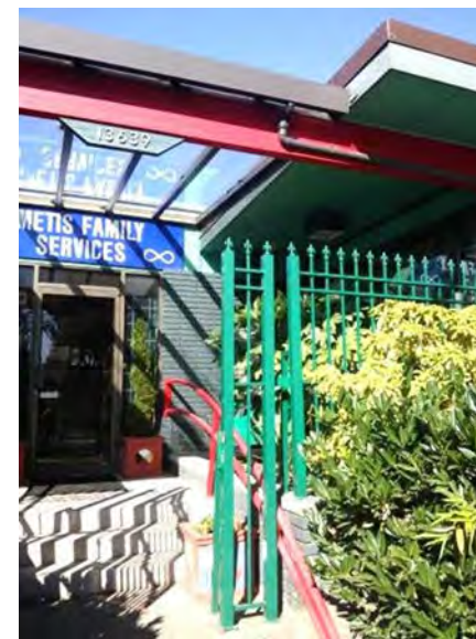
Enclosed breezeway area
