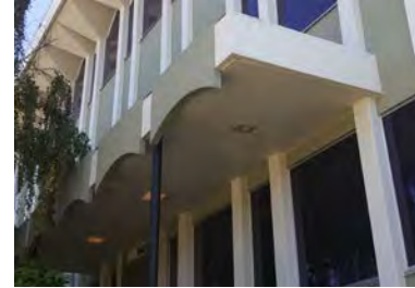
Concrete Canopy: Surrey
