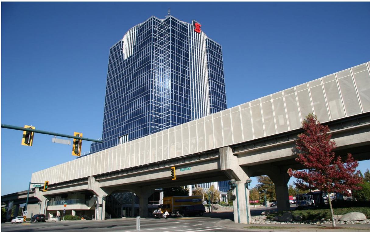
Gateway Office Tower, Surrey City Centre
