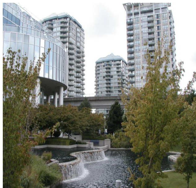
Gateway Office Tower public amenity space.
