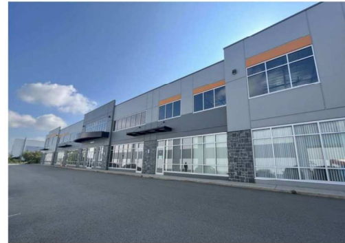
Commercial & Retail development located in 3237 190 St, Surrey
