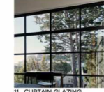
11 CURTAIN GLAZING Black powder coated Aluminium frame
