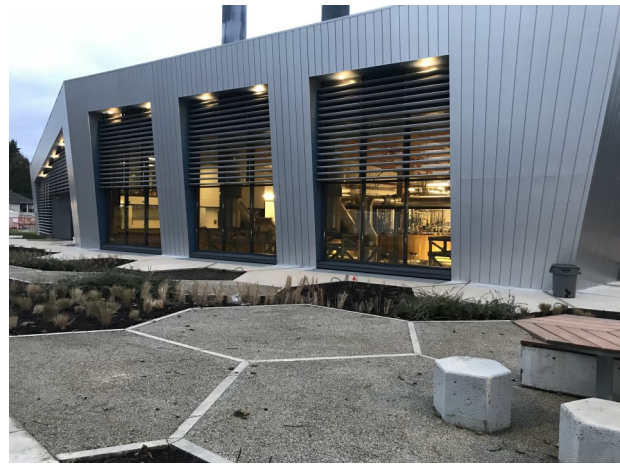
District Energy Centre
