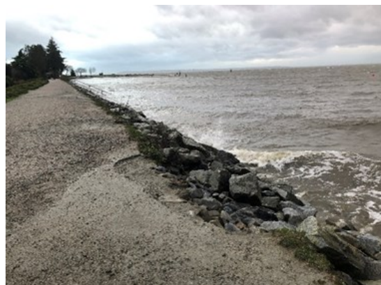
Crescent Beach Retaining Wall
