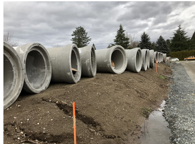
Sewer system installation
