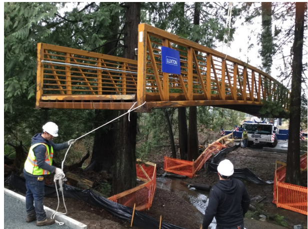
Hjorth Creek Bridge Installation
