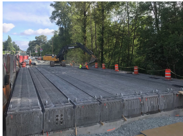
Bear Creek Bridge Replacement
