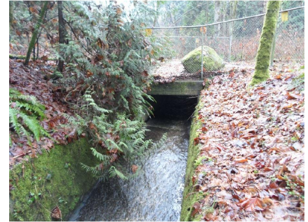
Photo 11: Bon Accord Creek concrete flume at downstream trail crossing
