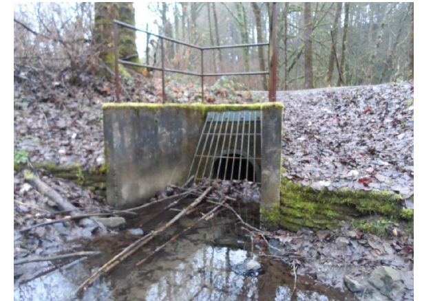
Photo 6: Culvert under trail to Bon Accord Creek
