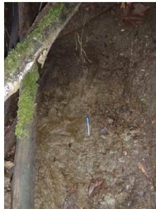
Photograph 9 Weathered soils atop competent till, Centre Ck. off Salisbury Dr.
