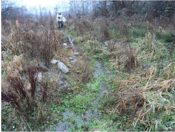
Photo 25: Outlet channel from stormwater pond
