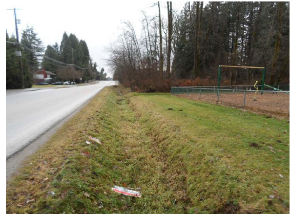
Photo 42: Drainage ditch along 156 th St. at Northview Park
