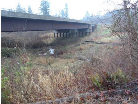
Photo 37: Potential planting areas on 184 th St. Creek next to Golden Ears Way
