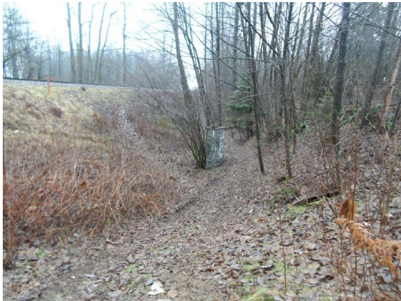
Photo 32: CV / pipe under railway
