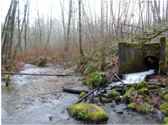
Photo 7: Culvert outlet for Bon Accord tributary
