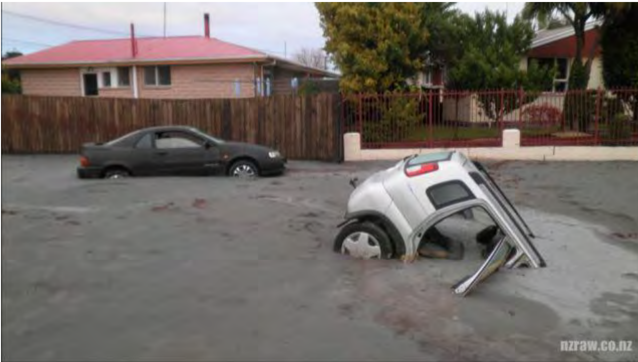
Liquefaction in Christchurch 2011 earthquake
