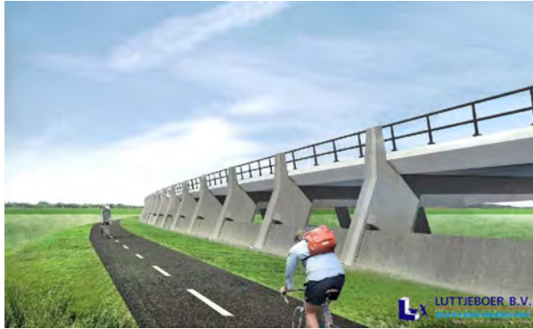
Elevated road above floodable area
