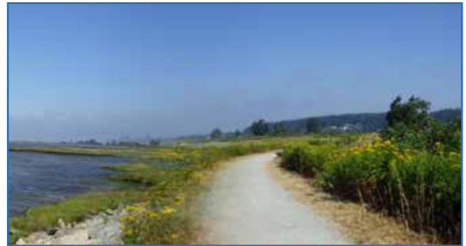
PHOTO: Colebrook Dyke Existing Crest
