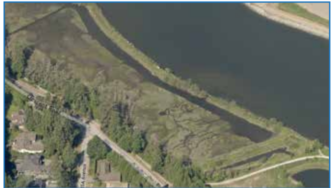
PHOTO: Location of the Stewart Farm Sanitary Pump Station on the south bank of the Nicomekl River
