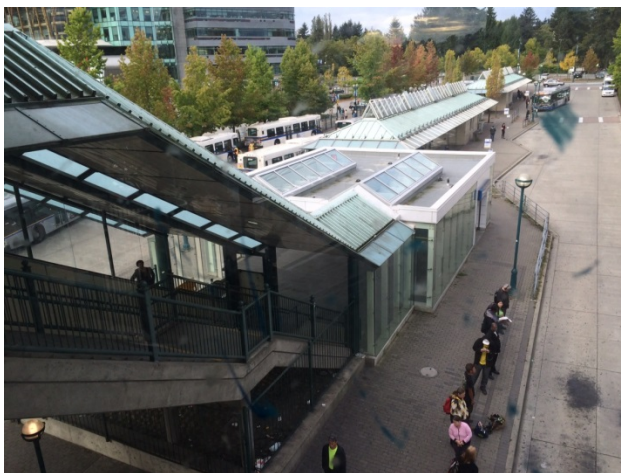
Current Day Surrey Central Exchange Looking West
