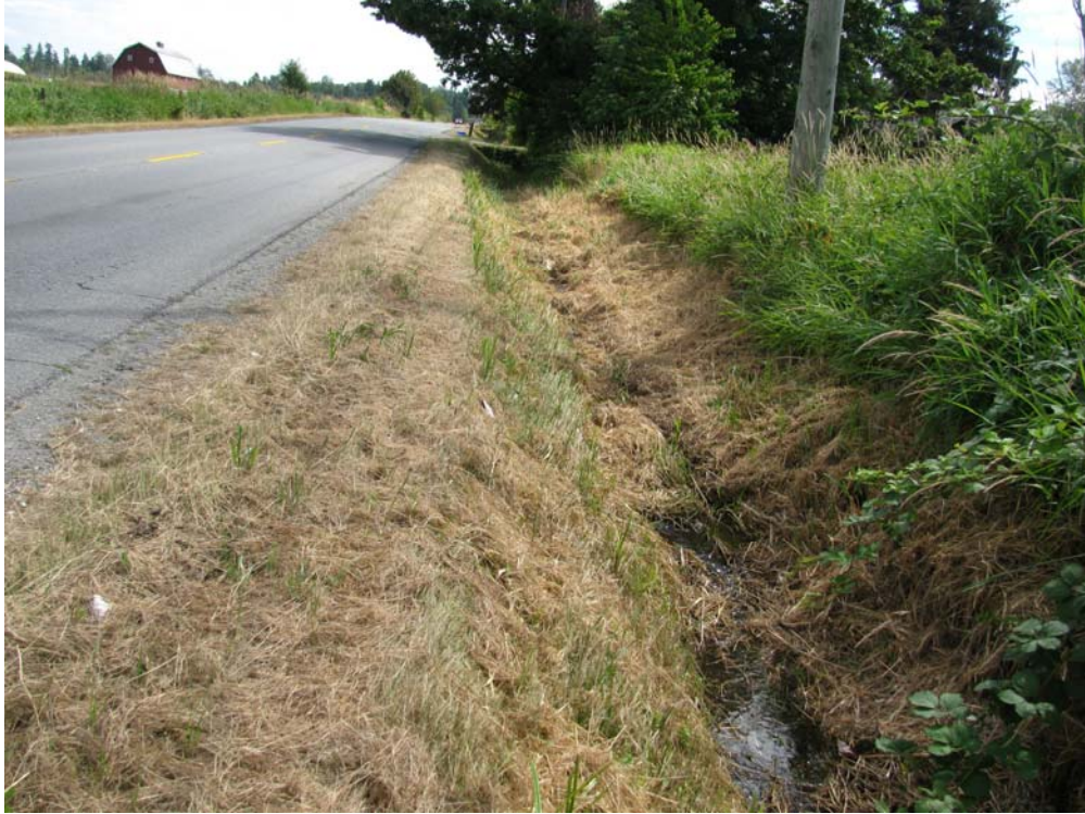
Typical lowland ditch along 80 th Avenue, east of 184 th Street (view east/upstream)
