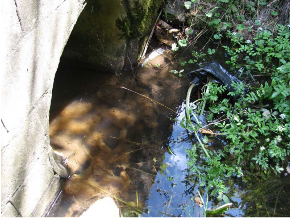
76 th Avenue Creek (view of upstream culvert headwall at 80 th Avenue)
