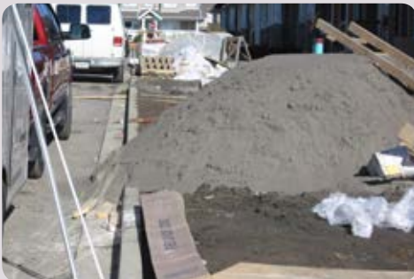
This image shows poor placement of an uncovered stockpile, no site perimeter controls, no surface erosion protection and dirt accumulated on the road and gutter.
