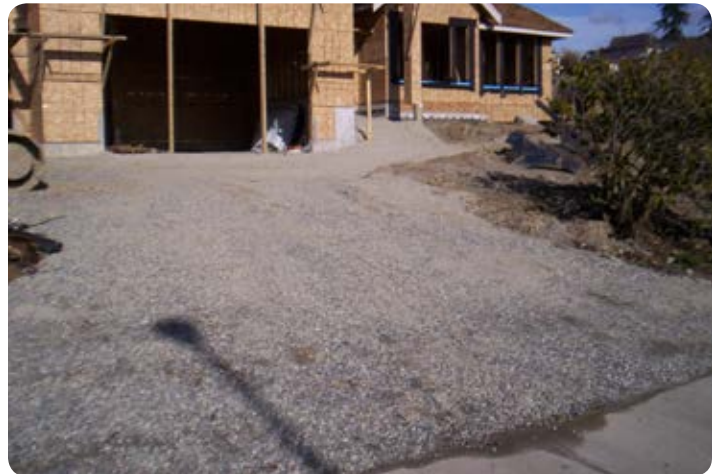
This angle of the same construction site shows that the builder has installed a gravel access pad for managed site access. The installed perimeter controls further act to restrict vehicles to this site access point, which that helps to keep the roads clean.
