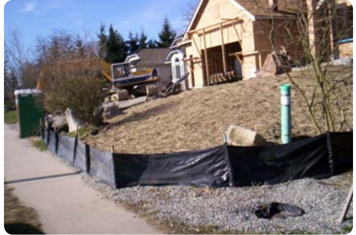
The above single family construction site shows a complete approach to site ESC management. There are perimeter controls, surface protection using straw, CB protection and the paved surfaces are clean.
