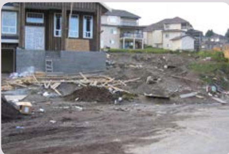
The site shows significant soil migration from the work area onto the road. No BMP's are present on this site and the road drainage is located under the material in front of the stockpile located in the middle of the image.
