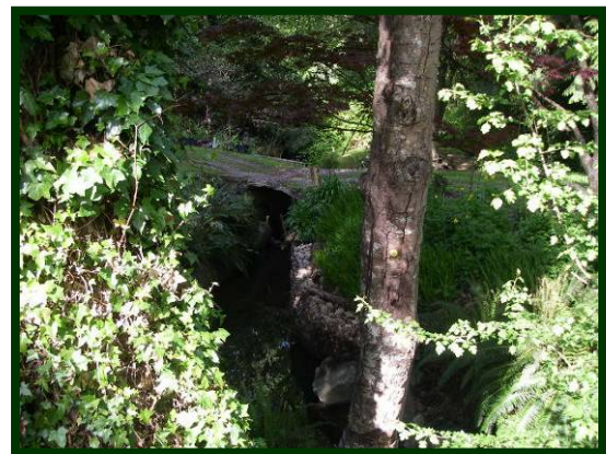
Photo 7.4: A Small Bridge Over Hyland Creek That May Require Upgrading
