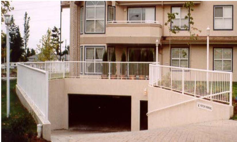
Gated ramp has good surveillance from adjacent units. Note lighting.
