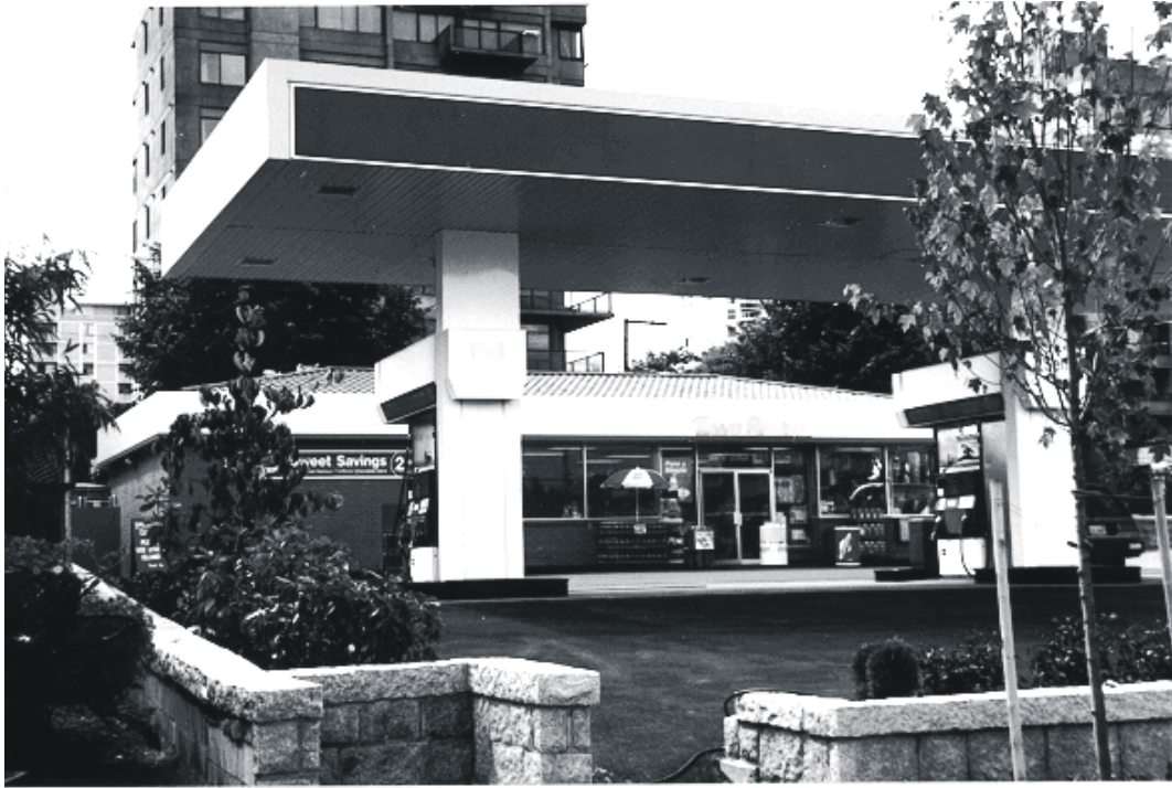
Fig. 10 Low walls and landscaping define the perimeter of the site and relate to the formal streetscape. Roof materials and form of the convenience store respond well to potential views from above. Good proportion between store, canopy and supporting structure.
