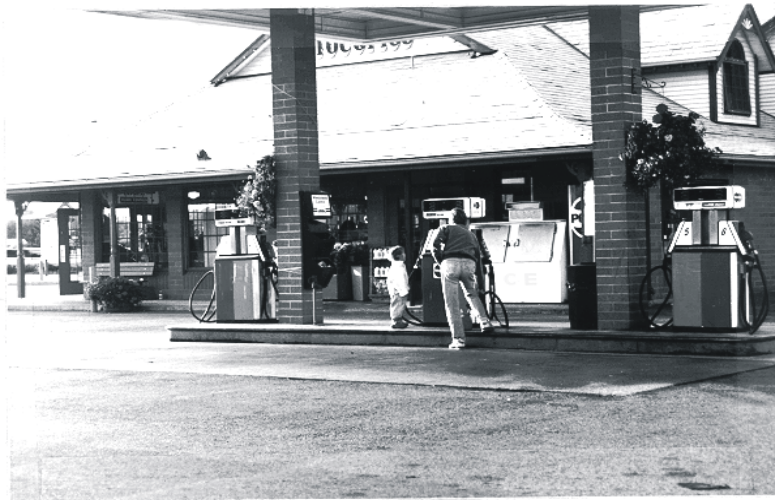
Fig. 2 Materials, proportion of the canopy supporting structure and the adjacent commercial building are compatible and reflect a residential character.
