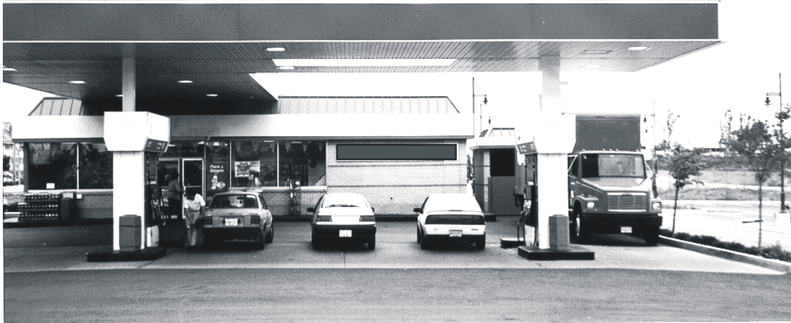
Fig. 11 Good linkage between canopy and the store. Skylights used to make the canopy appear lighter. Separation between gas pump islands may be reduced.
