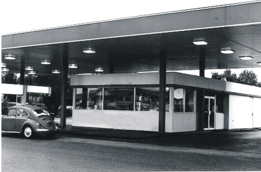
Fig. 8 The same materials are used in the canopy and the convenience store but the treatment of the facade is not carried around the building. The canopy appears too large compared to the convenience store.
