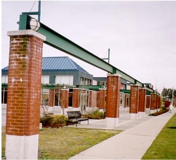
Brick pier and metal pergola defines semi-public space.
