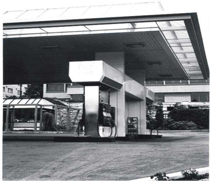
Fig. 7 Glass projection (skylight) at the edge of the canopy used to minimize fascia height and relate to commercial context. The architecture responds well to potential views from above.
