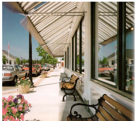
Extending interior space to street with benches, flowers, awnings, decorative paving and lamp standards.
