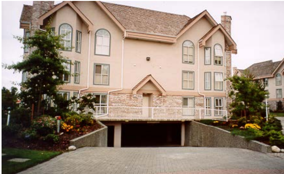
Note colour and texture on ramp, metal fencing along walkway, and overview from units above.
