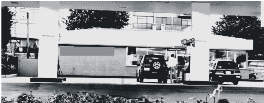
Fig. 3 Appropriate separation between gas pump islands. Proportions of the canopy support structure relate to the size of the canopy and the scale of the convenience store. Blank wall portion of the store presents some site security concerns.
