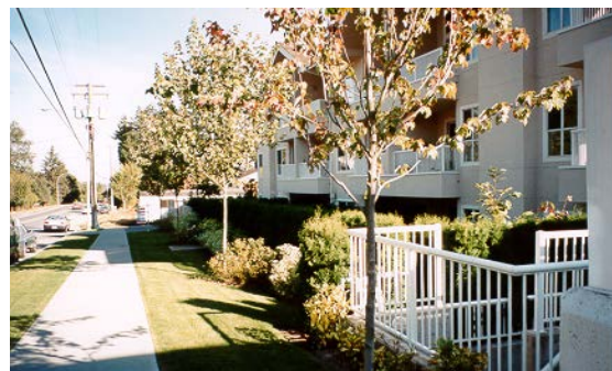
Enclose exit stairs to grade to prevent unwanted access.
