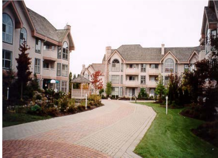
Clearly demarcated path to building entry marked by bollard lighting.
