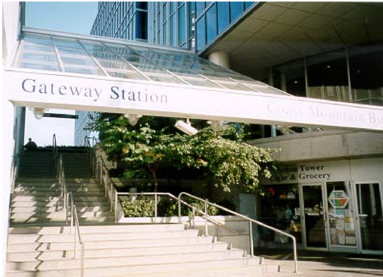
Note directional lighting at base of stair, but deep shadows near landscaped area.
