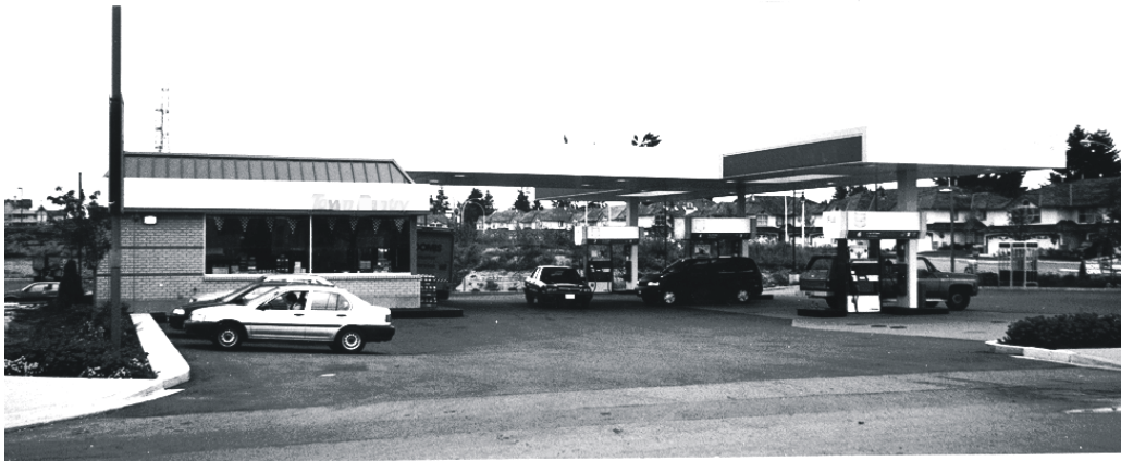
Fig. 12 Excessive width of entry driveway to the site could have been avoided. Opportunities exist to bridge the gap in continuity of the sidewalk by using landscaping to screen the parking area.
