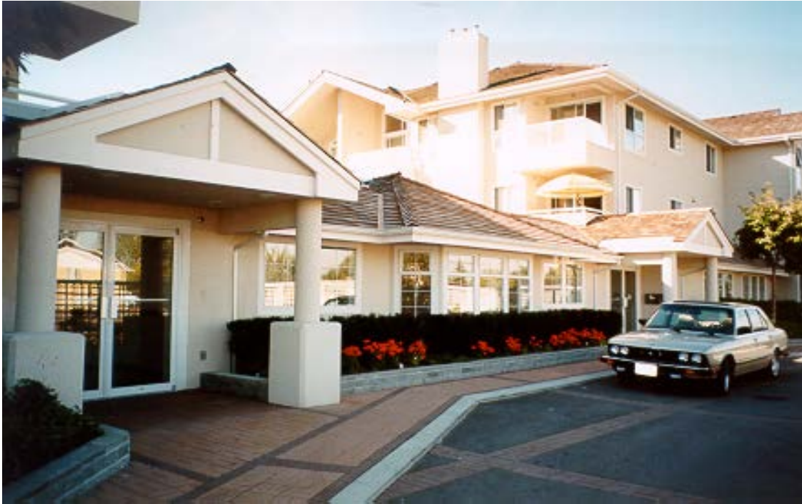
Entry to amenity building is obvious and well glazed, both providing and receiving good surveillance.
