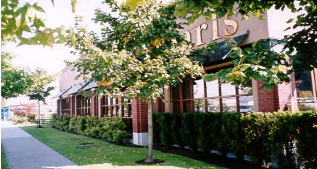
Combination of transparent and opaque glazing to maximize perception of surveillance along sidewalk.
