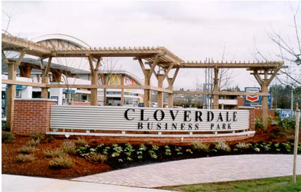
CPTED principles of hierarchy of space used to define territoriality in commercial developments.
