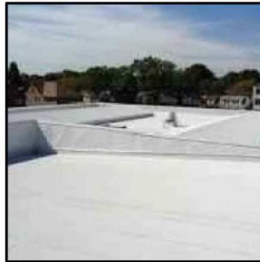
7 Soprema Soprastar roofing by Soprema with RSI .82
