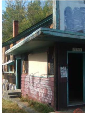
Note the wrap around shed roof, that extends out less towards the side door. The other side is the same.
