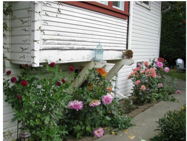
Missing bracket on south elevation
