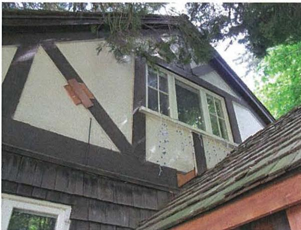
South elevation: half-timbering (to be repaired),
