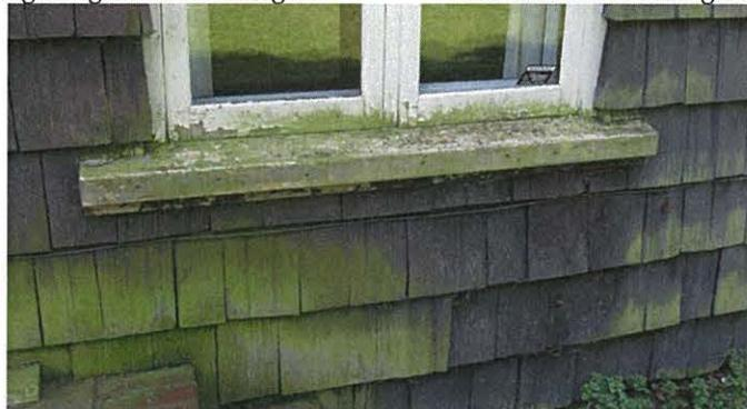
North elevation window frame and sill showing deterioration
