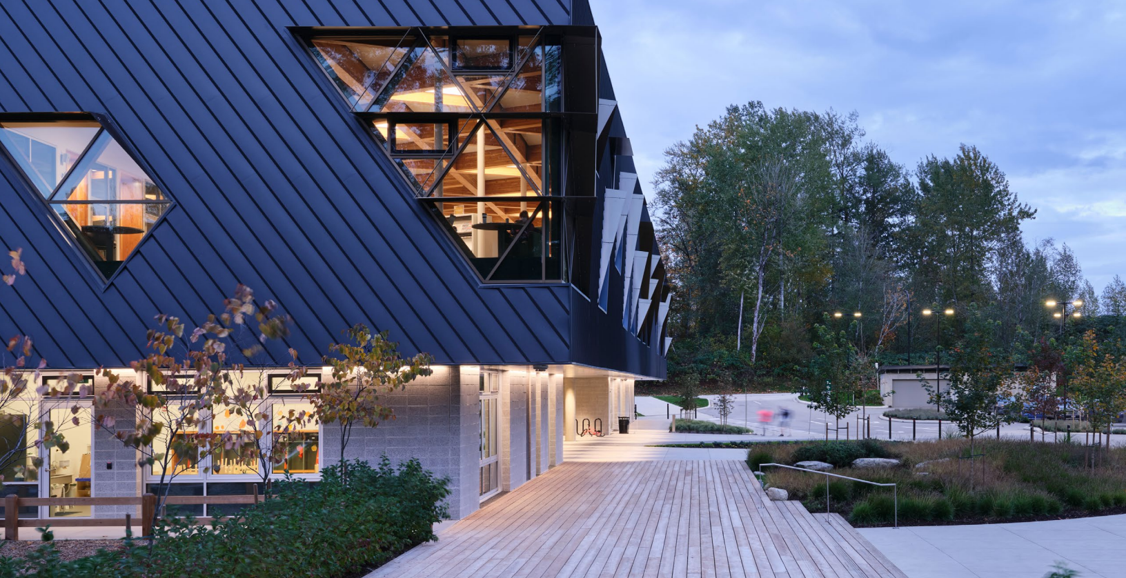
Clayton Community Centre - North America's first Passive House certified community centre (source: @andrewdoranphoto, courtesy of hcma)
