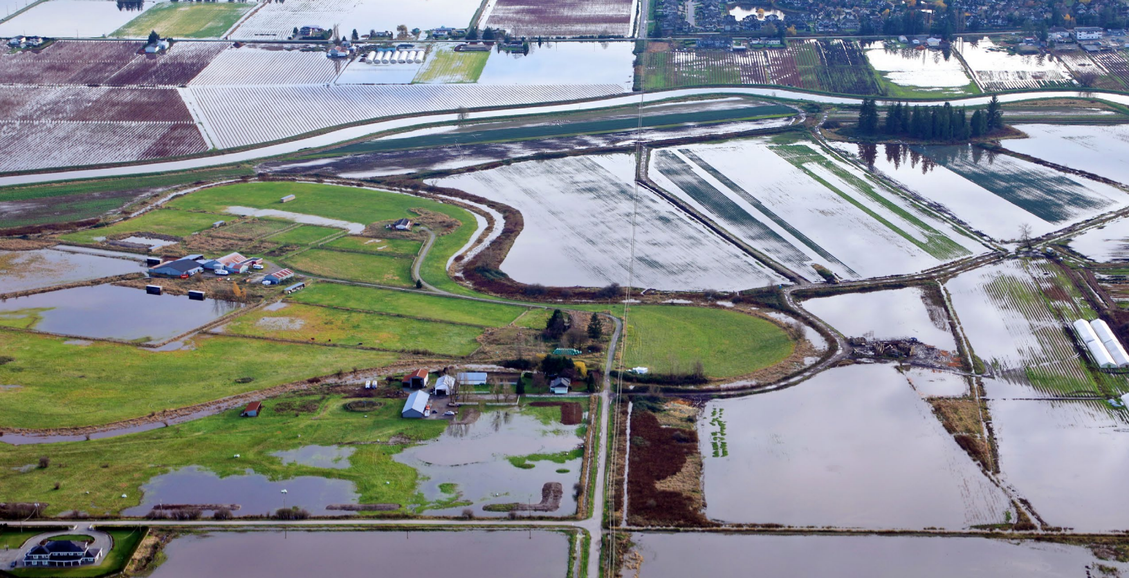
Flooding in South Surrey after the November 2021 atmospheric river event (source: City of Surrey)
