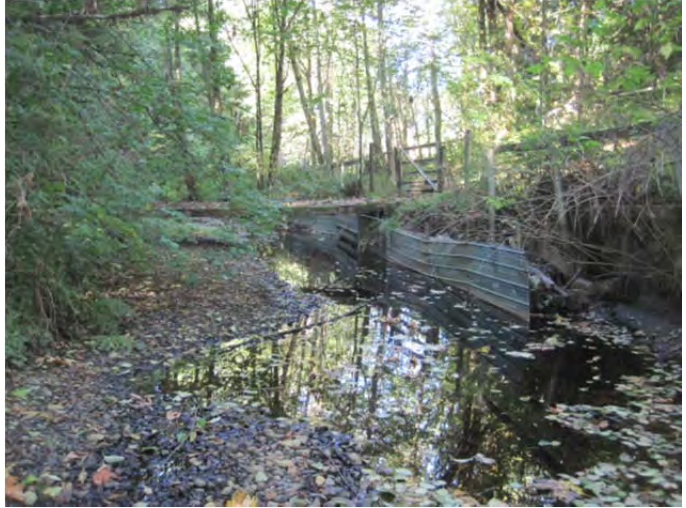
Photograph 10. ↑ Looking upstream from AND-03 sample location from a footbridge across the stream, towards bank armouring along left bank (October 3, 2012).
