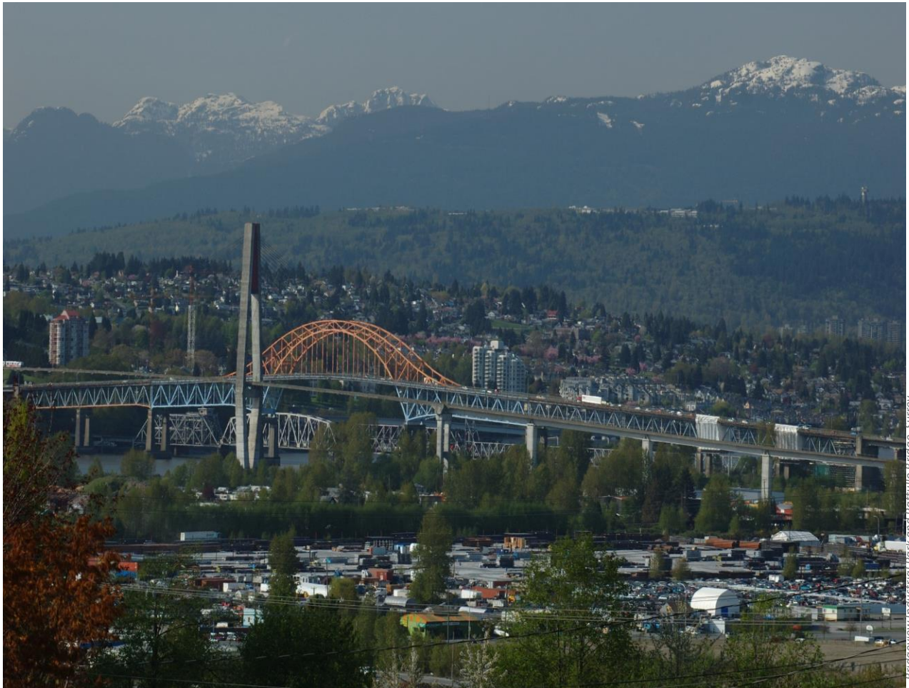
Bridgeview Industrial Park and Pattullo Bridge, Surrey.
