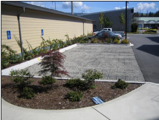
Reinforced Clean Crushed Gravel
