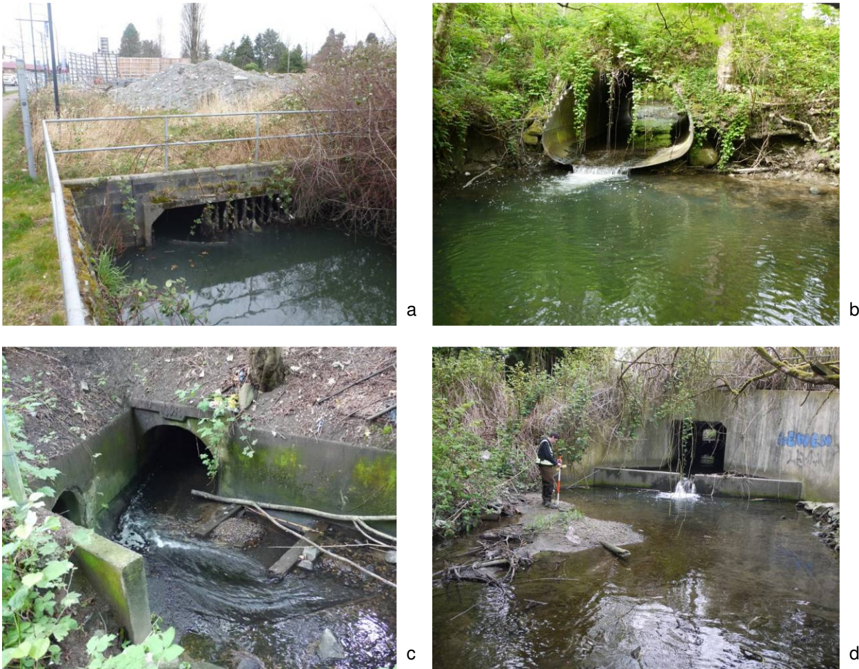
Figure C-21: Fish passage issues in Quibble Creek: (a) is the upper extent of Quibble Creek mainstem near 100 Ave; (b) culvert barrier to juvenile fish under low summer flows at 94A Ave; (c) passable culvert under Fraser Highway (upstream end with baffles); (d) culvert outlet control downstream of Fraser Highway may restrict fish movement under lower flows.
