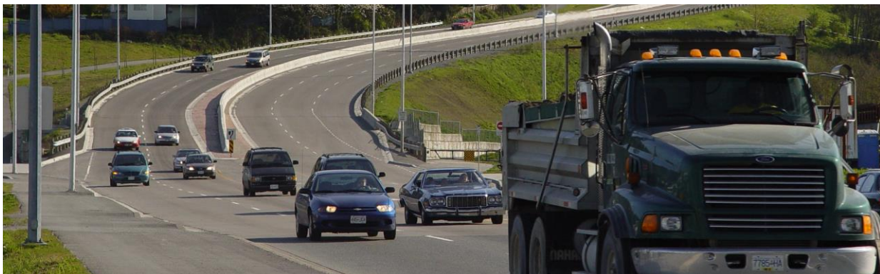
Scott Road transportation corridor, Surrey.
