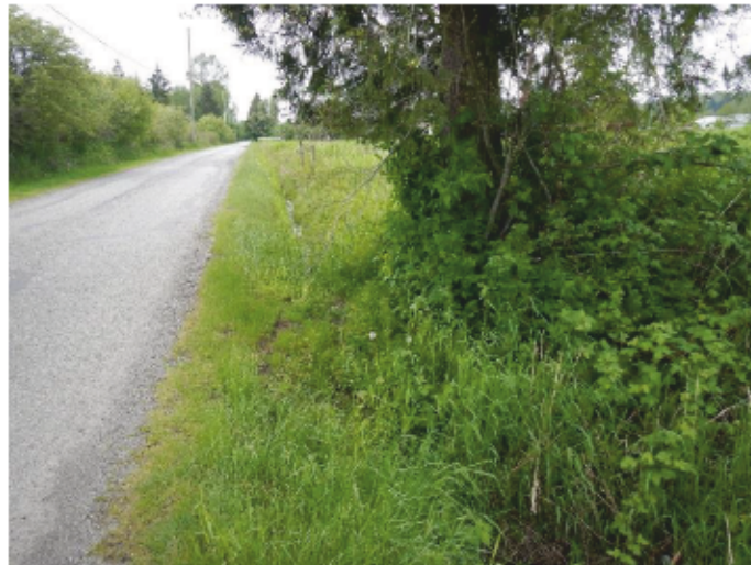
Culvert inlet (top left), outlet of upstream culvert (top right), upstream of inlet (bottom)
