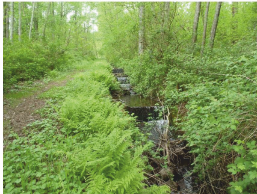
Photo 7: Class A(O) Watercourse. Upstream view of Watercourse 7 with steep, modified step-pool habitat with concrete weirs creating barriers to fish passage.
