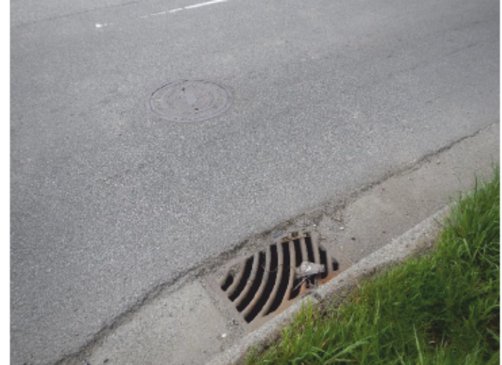
Looking upstream along old ditch alignment (top left), looking downstream of old ditch alignment (top right), catchbasin on HWY 15 suggesting piped storm system (bottom right), ditch may have been filled to provide noise abatement berm for residents (bottom left)
