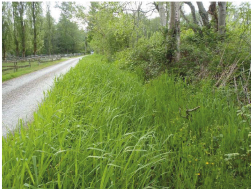
Photo 23: Class C Watercourse. West (Upstream) view of Watercourse 6 near concrete culvert leading to Watercourse 9.
