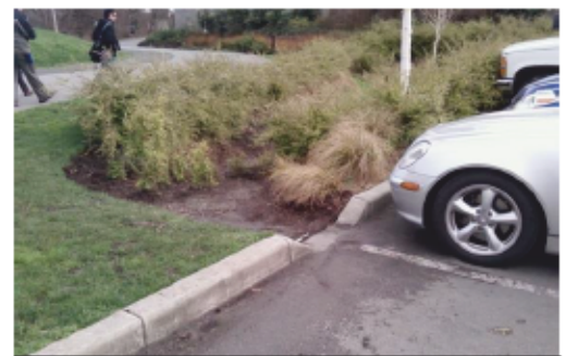
Rain garden adjacent to parking lot.
