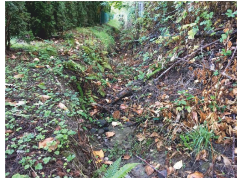
Photo 12: Class B Watercourse. Upstream view of Watercourse 3. Well defined, scoured channel.
