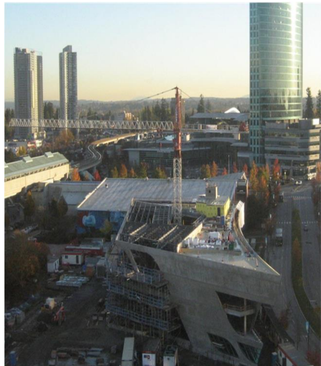
Surrey City Centre Library, under construction.
