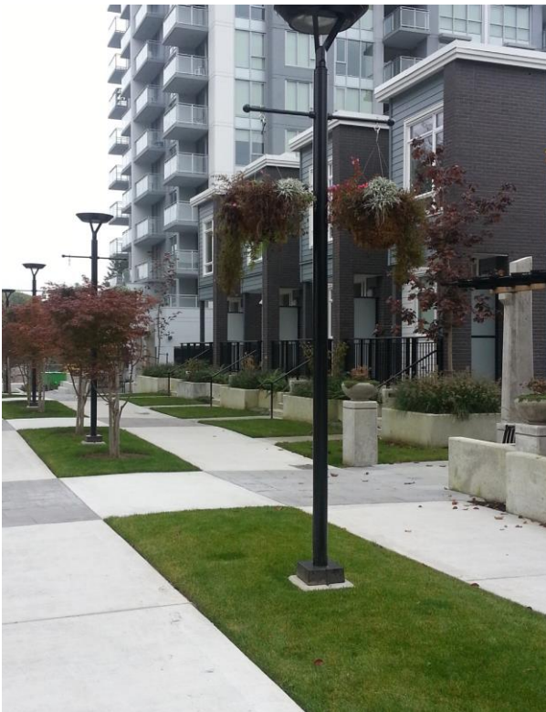
WestStone Development, Surrey City Centre; public infrastructure installation.
