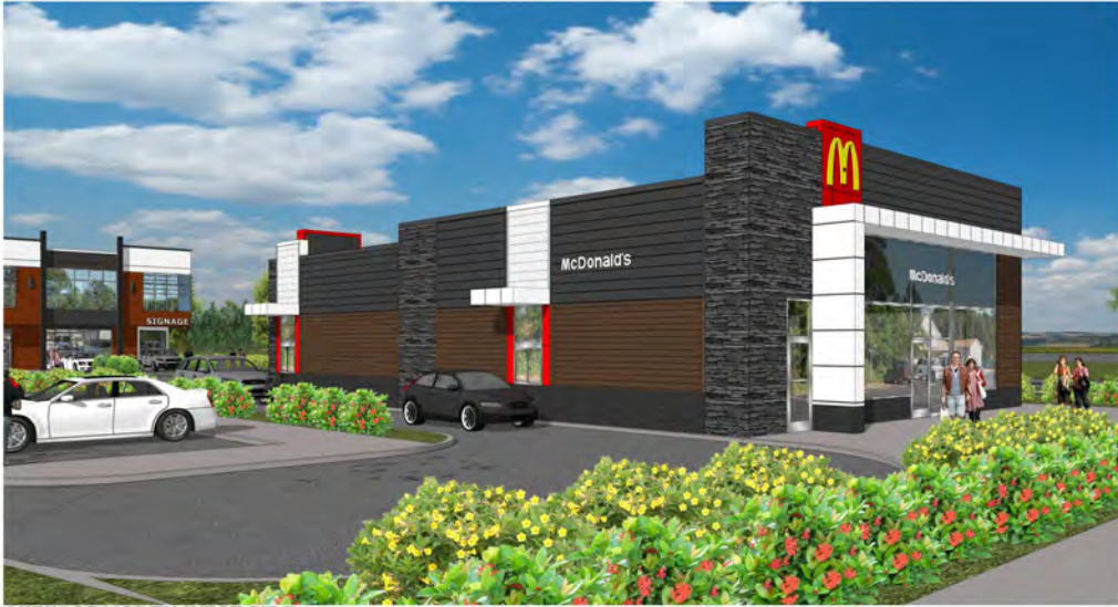
VIEW OF NORTH WEST SIDE
