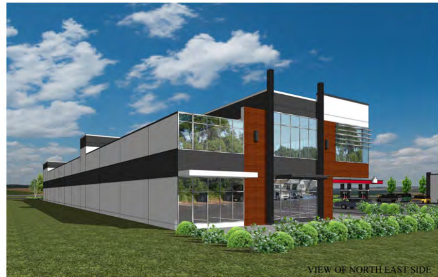
VIEW OF NORTH EAST SIDE
