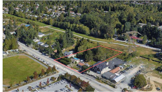
EXISTING AERIAL VIEW
