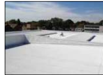
SOPREMA SPOPRASTAR HIGH ALBEDO ROOF WITH SRI VALUE OF .82
