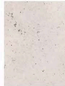
CONCRETE WALL COLOUR: 'CLEAR SEALER'
