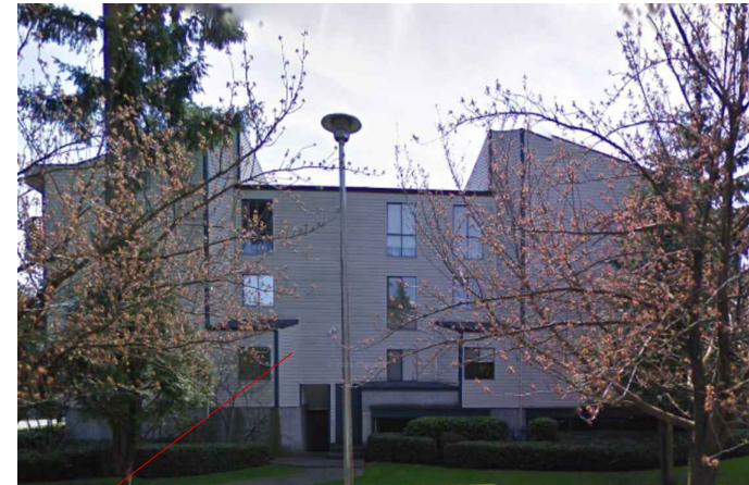
Existing Building from 100 Avenue
