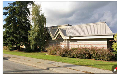
3. GROCERY STORE NW OF PROJECT SITE
