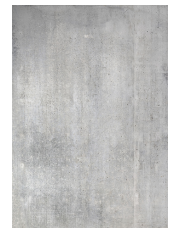
CONCRETE COLUMNS AND WALLS
