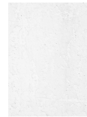
PAINTED CONCRETE SOFFIT
