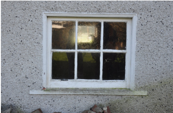
Typical multi-pane fixed (alternatively, casement or awning configuration) window with true divided lights on basement level.
