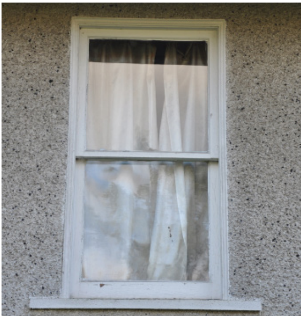
Typical double-hung wood sash assembly
