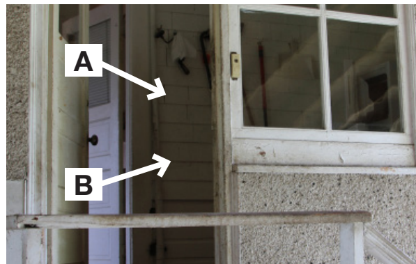
Localized areas showing surviving original wood cladding: cedar shingles (A) and shiplap siding (B).
