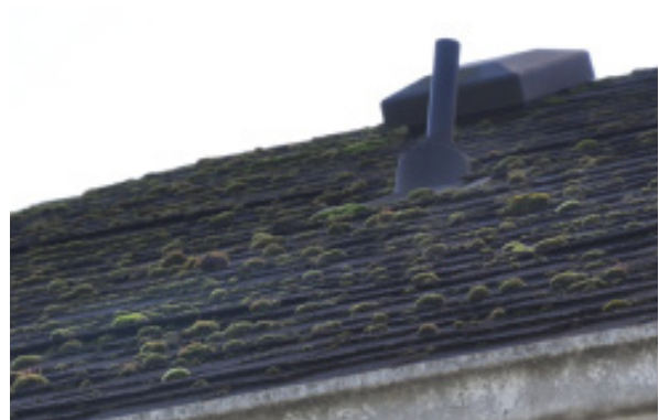
Existing condition of replacement asphalt roof shingles facing south (left) and north (right). Note heavy biological growth on roof cladding facing north as a result of moisture saturation caused by minimal sun exposure.
