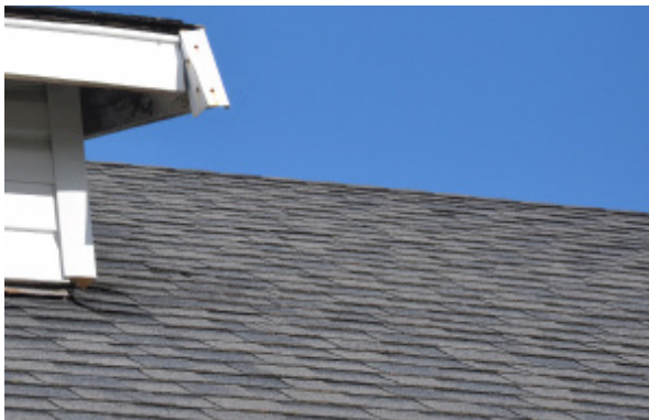
Existing condition of replacement asphalt roof shingles facing south (left) and north (right). Note heavy biological growth on roof cladding facing north as a result of moisture saturation caused by minimal sun exposure.
