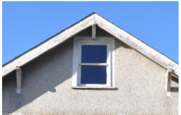
Double-hung wood sash assembly at rear gable wall (attic).
