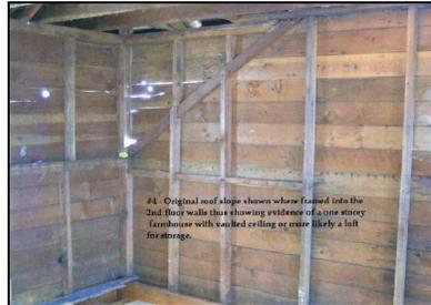
The gable ends also show the slope of the original roofline. At some point (probably before the Baron took ownership as the spacing of studs and rafters are 24 -30" apart) the owner extended the walls for a second storey and built a new roof complete with dormers.
