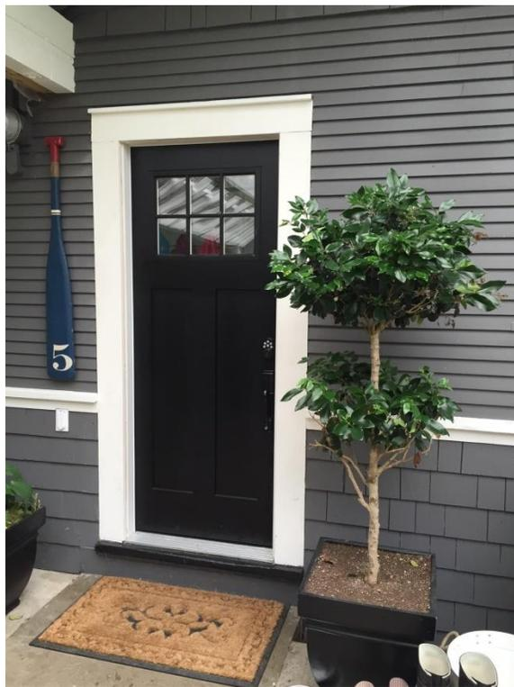
Combination of lapped and shingle cladding
