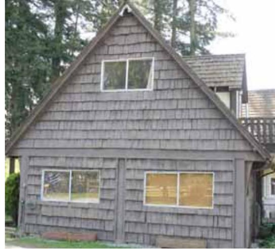
Non-original metal windows on the northeastern elevation, which should be replaced with more historically appropriate wooden frames and sashes
