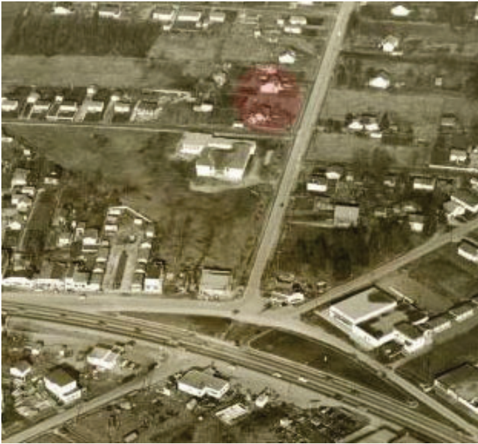
Figure 32: 1953 Aerial photo of King George Highway and Grosvenor Road with 13667 & 13683 in red ellipse (Cosmos)
