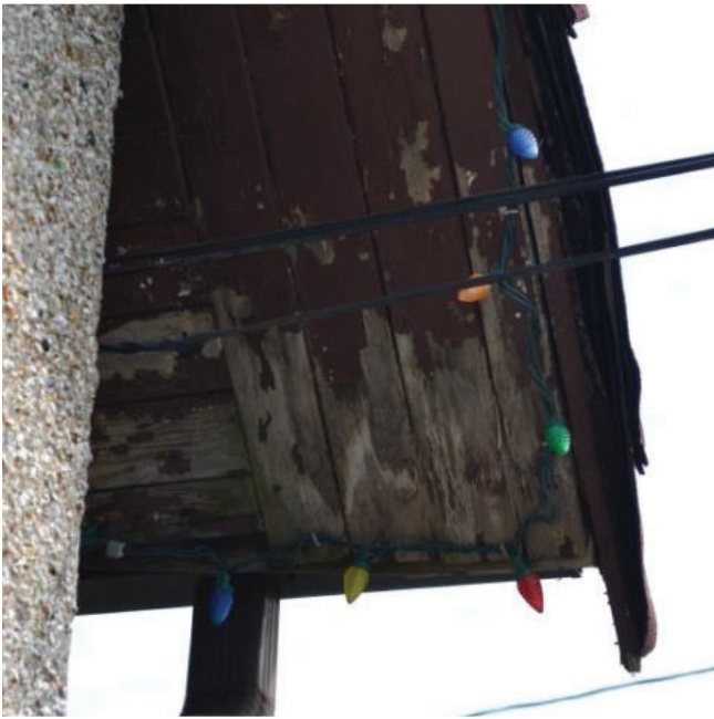
Figure 41: Wood board open soffit
