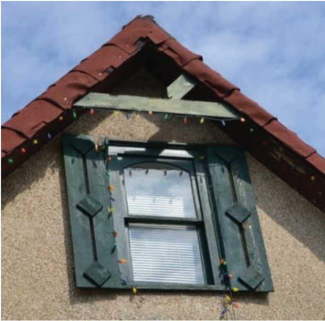
Figure 36: Architectural truss at front gable end
