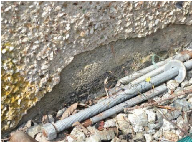
Figure 45: Parging beneath stucco
