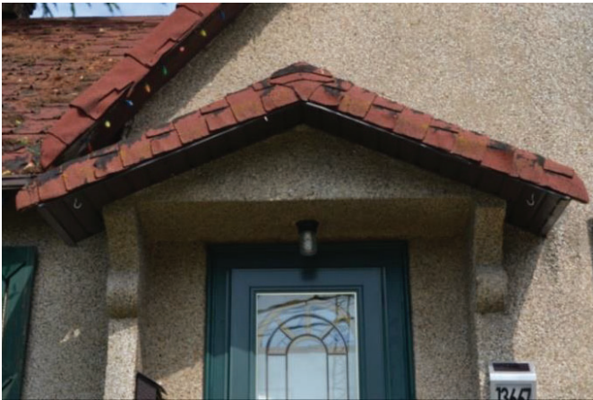
Figure 36: Architectural truss at front gable end
