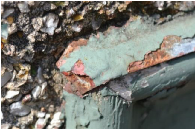
Figure 46: Added metal flashing and wood trim
