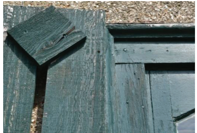
Figure 47: Decorative frame added on top of stucco
