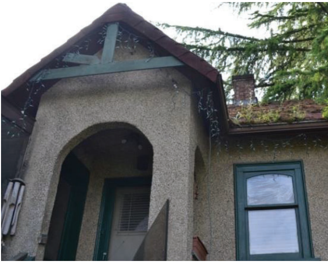
Figure 43: Arched back entrance with architectural truss
