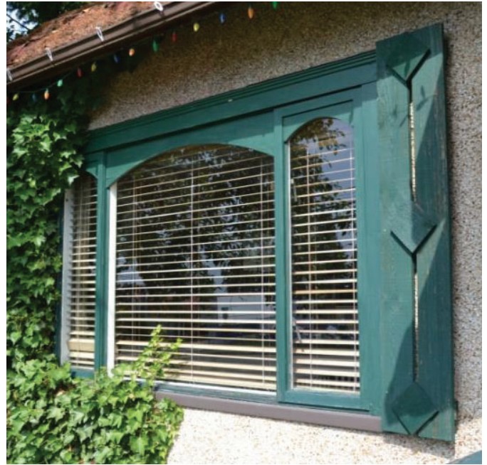
Figure 39: Internal arch living room windows
