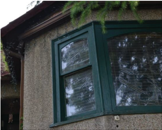
Figure 42: Double-hung window with upper internal arch
