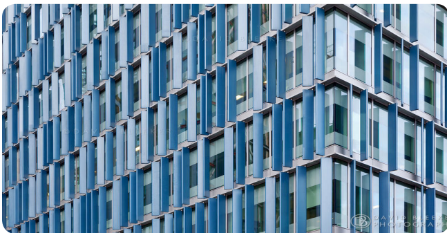
Vertical shading devices can be added to a building's west facade to shade from hot afternoon sun, and can act as privacy screens between exterior balconies.
