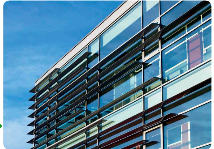
Horizontal shading devices can be added to the south and east facades where balconies are absent, or where they do not provide adequate summer shading.
