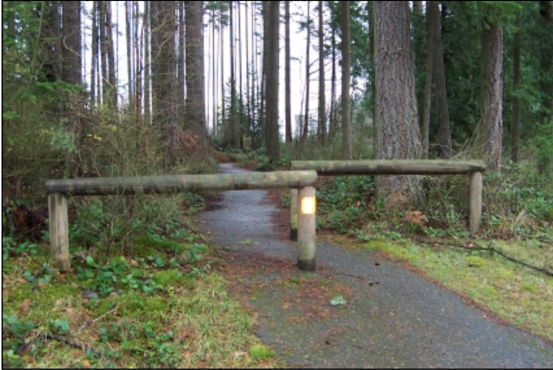
Figure 17. Wooden fencing at the entrance to Trail #2
