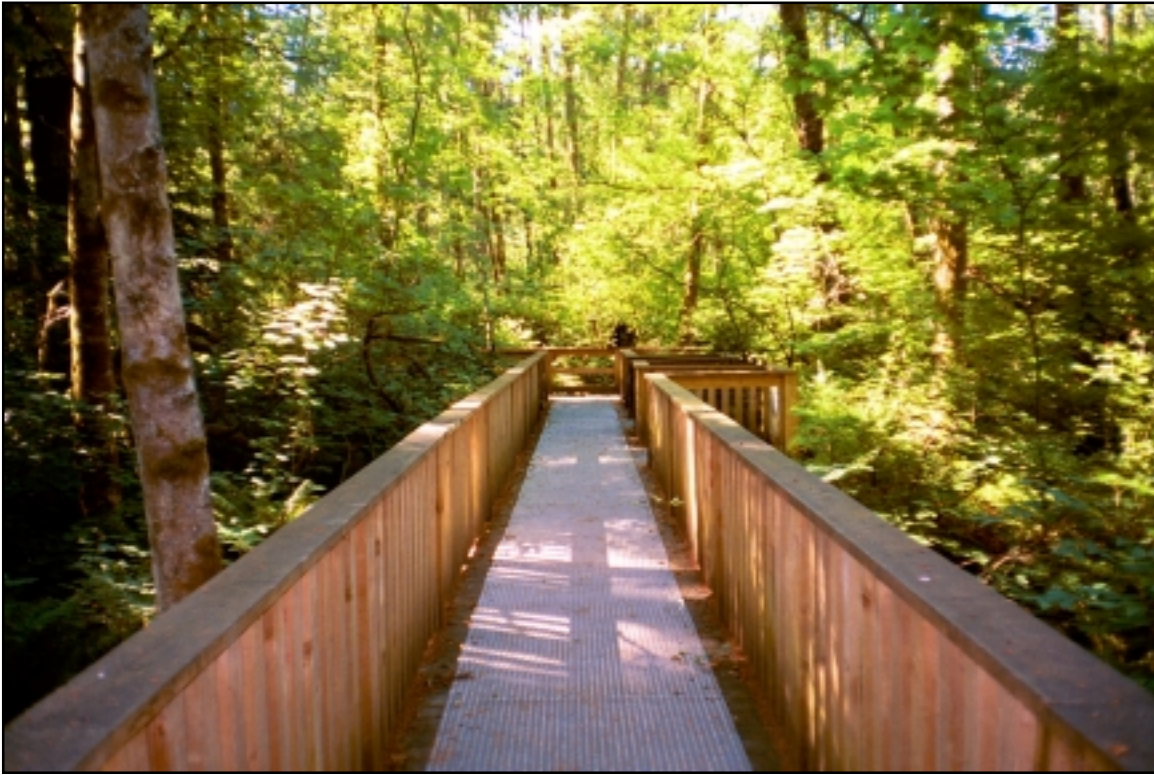
Figure 6. Boardwalk constructed along the Wally Ross Trail
