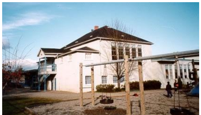
Figure 2: Tynehead Elementary School - West Wing (est. 2000)
