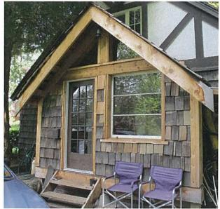
South elevation entryway addition: door, window, bargeboards, cornerboards and shingles should more closely match the remainder of the cottage
