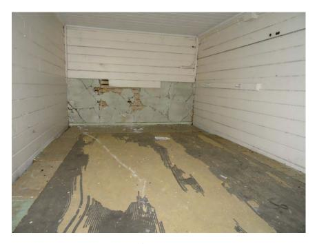
This damaged wall at the entry foyer allowed us determine the wall structure. The walls are framed using 2x4 most likely rough cut lumber at 16" o.c. which is also the spacing of the ceiling jooists.
