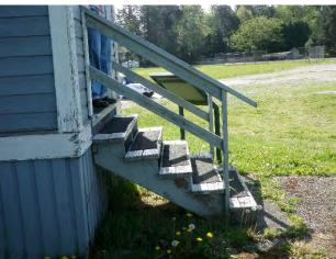
The access stairs to the school building were adequately constructed; however the treads and stringers are well aged and should be replaced. The railings do not comply with the current building code.
