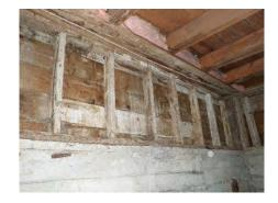
The original floor joists were rough cut 2x6 at 24" o.c. The joists extend to the exterior sheathing with more than adequate seats on the 4" deep top plate pf the pony wall (see next photo). It appears that during the last renovations some joist may have been damanged and were doubled and also some new joists were added.
