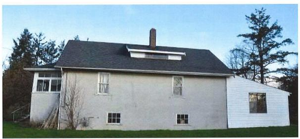
South elevation showing primary front-gabled wood-frame roof structure, shed dormer, interior brick chimney, hipped-roof (verandah), and shed-roof (rear extension, not original).
