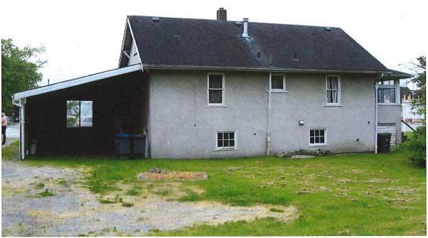
Side (north) elevation of Main Residence, showing later shed-roof extension to the rear (left) and front verandah (right). Note unifrm settlement at northwest corner of front verandah.
