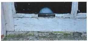
Photo showing typical deterioration of existing wood sashes.
