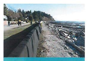
Temporary concrete barriers put up after March 10th, 2016 storm damage.
